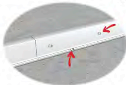
MEASURE & MARK POSITION OF INTERMEDIATE PORTAL FRAMES
