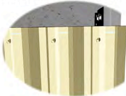
MARK A CHALK LINE WITH A SLIGHT DOWNWARD SLOPE TOWARDS DOWNPIPE END
