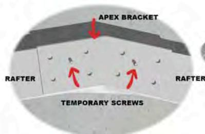
MEASURE AND ADJUST RAFTER TO EQUAL "RAFT DIST"
